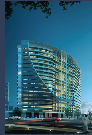
The V Tower
